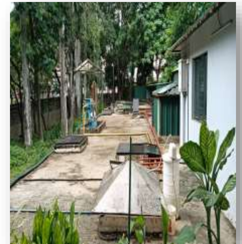
Sewage Treatment Plant
